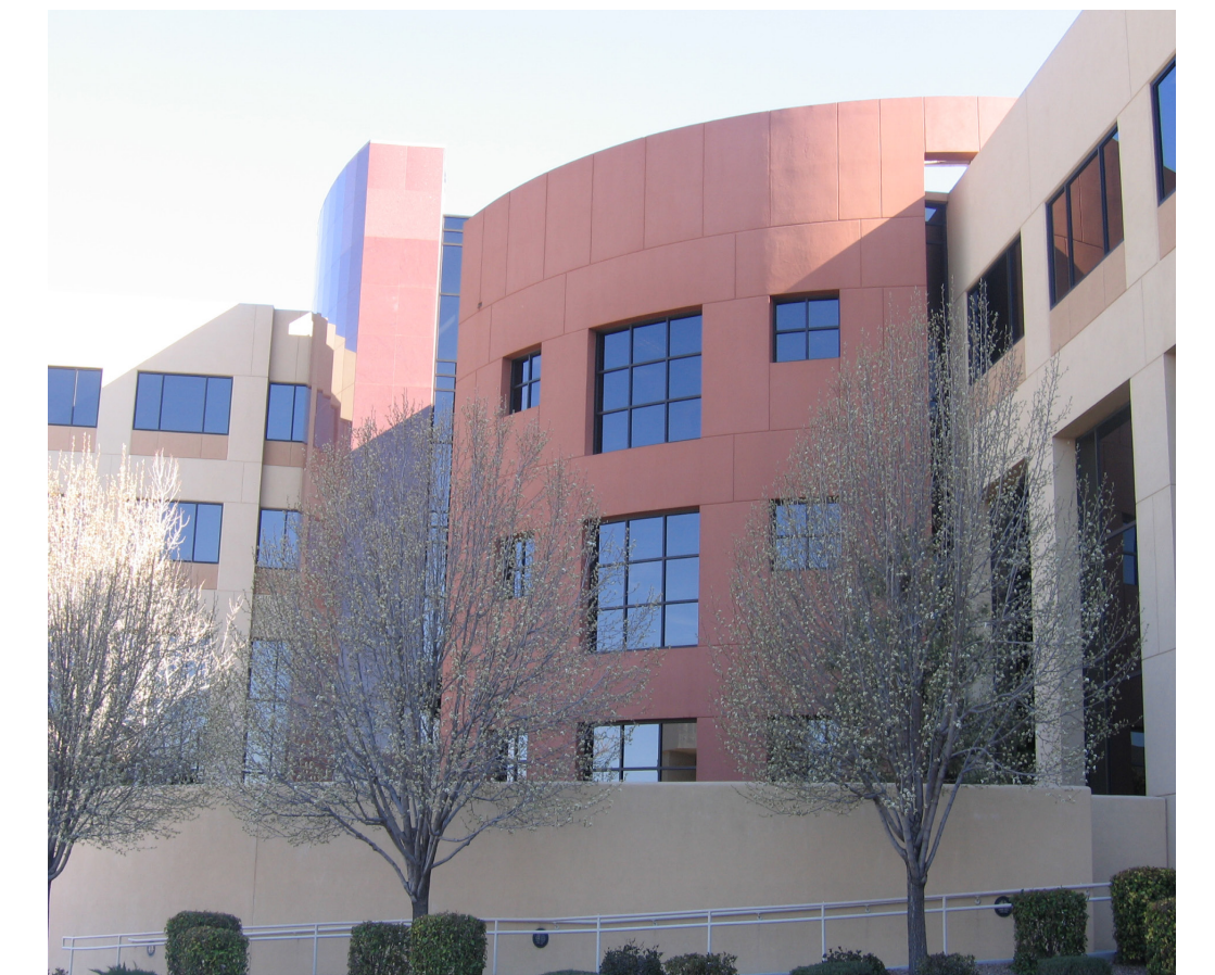
Altura Office Building
