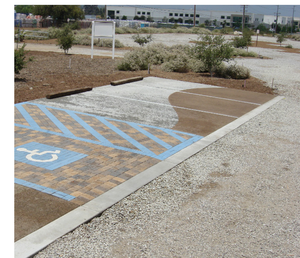
Pervious Surface Materials on Parking Lot
