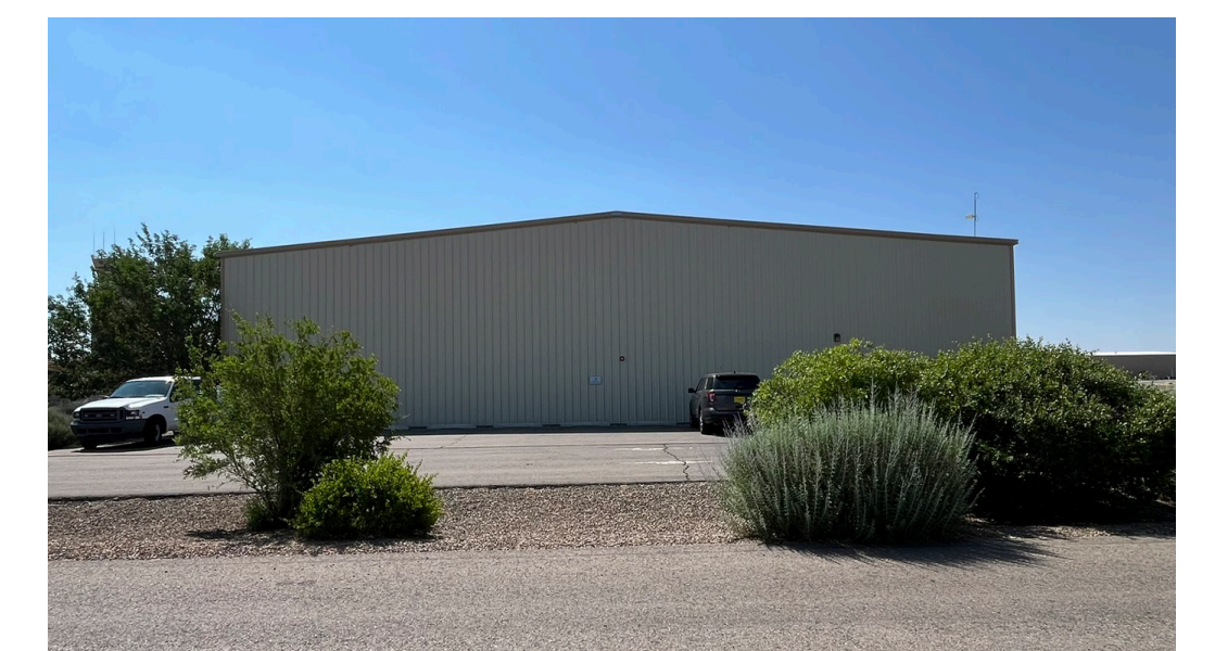
Existing Stormwater Control from an Executive Hangar
