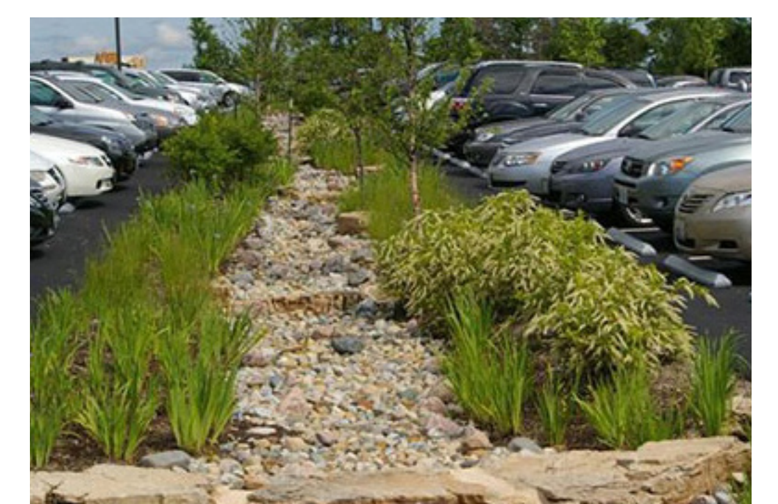
Parking Island Stormwater Control Area
