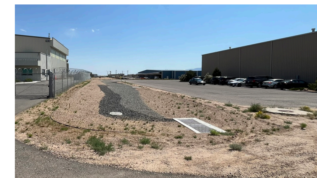
Existing Stormwater Control at NM State Police Hangar
