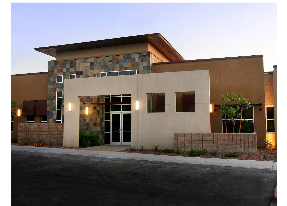
Red Rock Office Building
